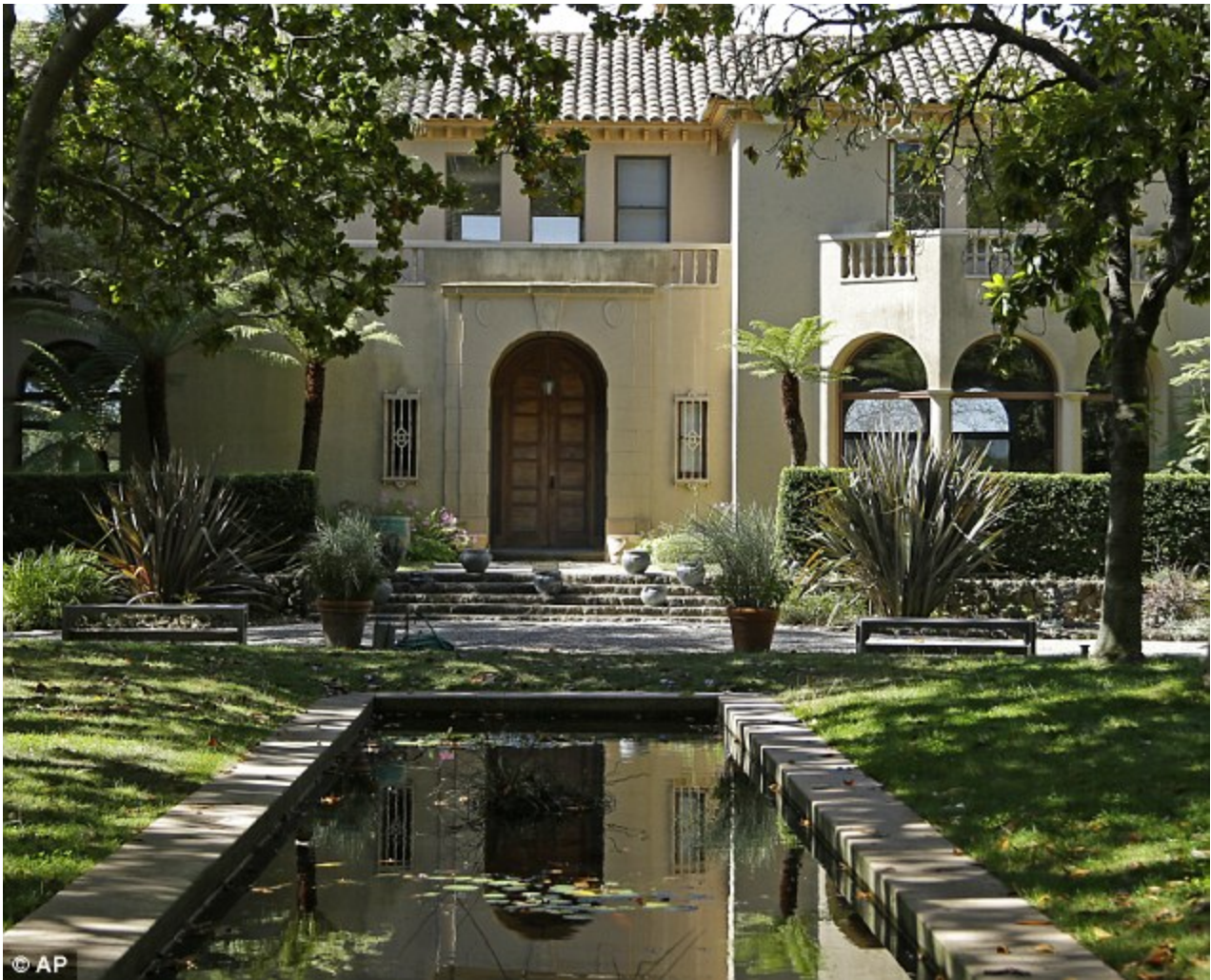
University of California prepares to repair and renovate this 13,269-square-foot mansion, the Blake House, that for decades housed past University presidents. Located in East Bay hills not far from the Berkeley campus, house has been vacant since 2008 and declared uninhabitable following years of neglect
